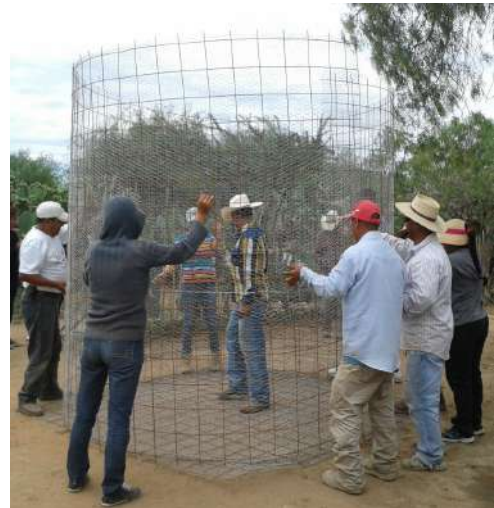
Figure 3.8 — A group constructing a cistern hold their reinforcement cylinder and base.
