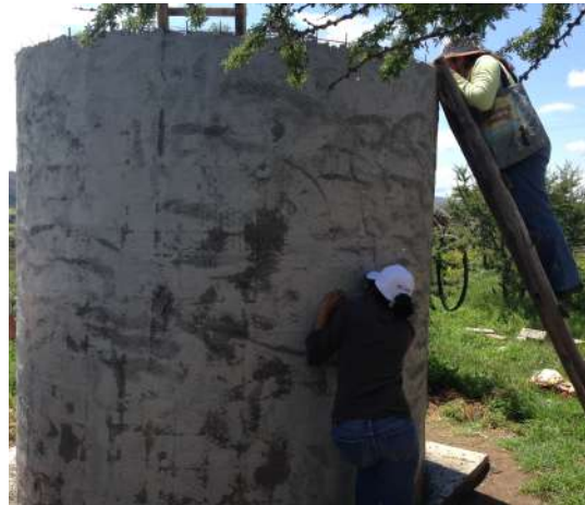
Figure 3.10 — An in-process cistern with completed wall and base.
