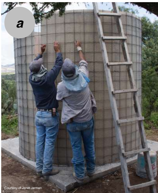
Figure 3.11 — An in-process cistern with completed base has almost all of its formwork attached. The same cistern is shown from the (a) outside and (b) inside.
