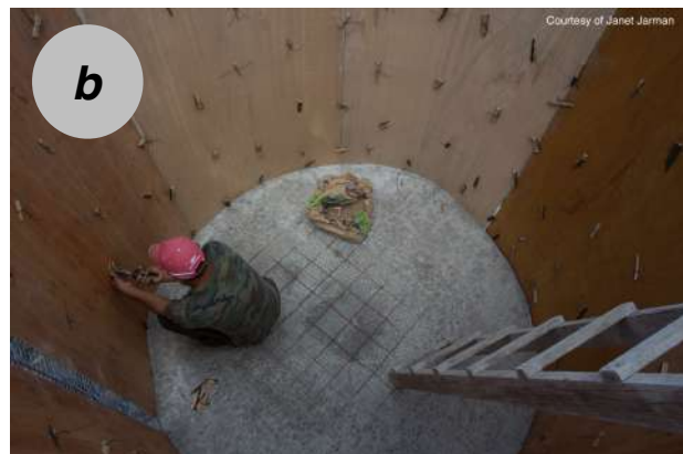
Figure 3.11 — An in-process cistern with completed base has almost all of its formwork attached. The same cistern is shown from the (a) outside and (b) inside.
