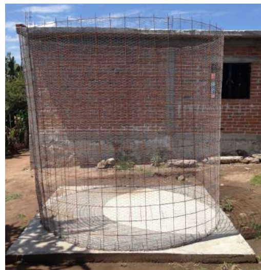
Figure 3.9 — The reinforcement mesh cylinder sticks up from a completed concrete base.
