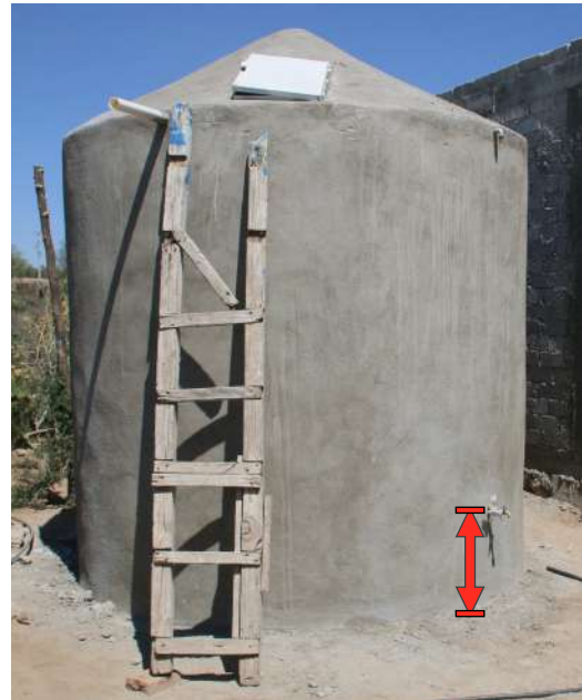
Figure 3.2 — Height of tap from ground
